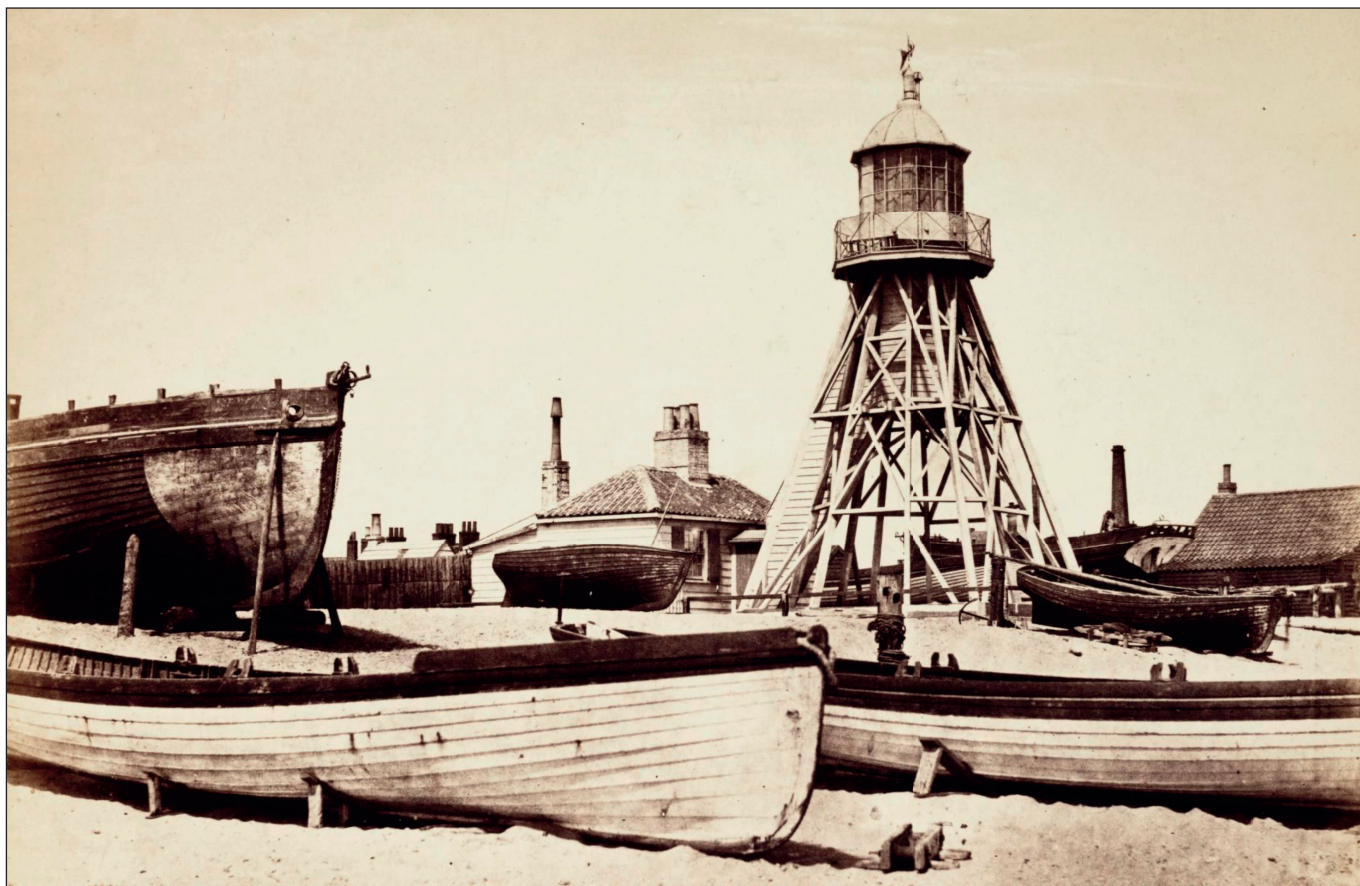
ABOVE: The Lowestoft Low light (4) of 1730, an essentially timber framework, with an enclosed lantern of square-pane glass. BELOW: The Lowestoft Low Light (5) of 1866 made of cast and wrought iron, its lantern glass having rhomboid (diamond) geometry.
